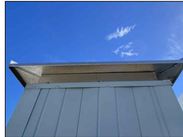
P15 DETAIL VIEW OF S.S. CAP
