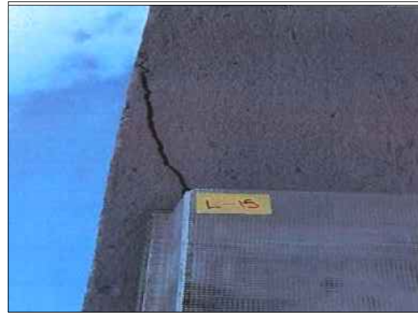
P4 ROOF COLUMN REPAIR
