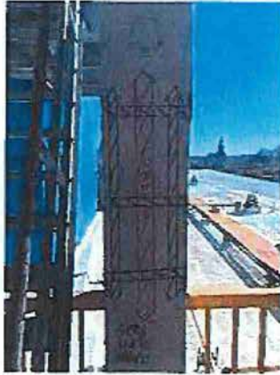
Loc. 10 Typical Rebar Pattern
