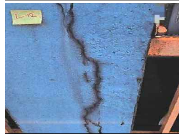
P3 ROOF COLUMN REPAIR
