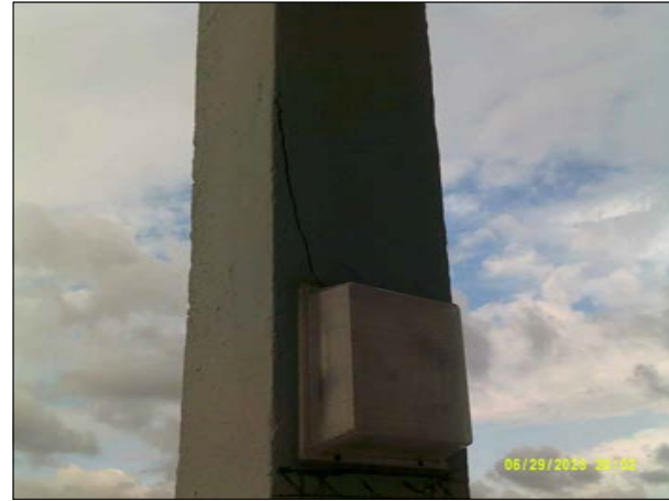
P1 ROOF COLUMN REPAIR
