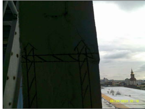
P2 ROOF COLUMN REPAIR
