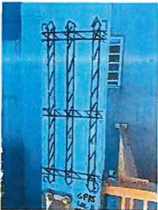
Loc. 11 Typical Rebar Pattern
