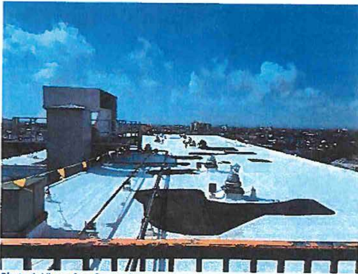
Photo 4: View of roofing replacement.
