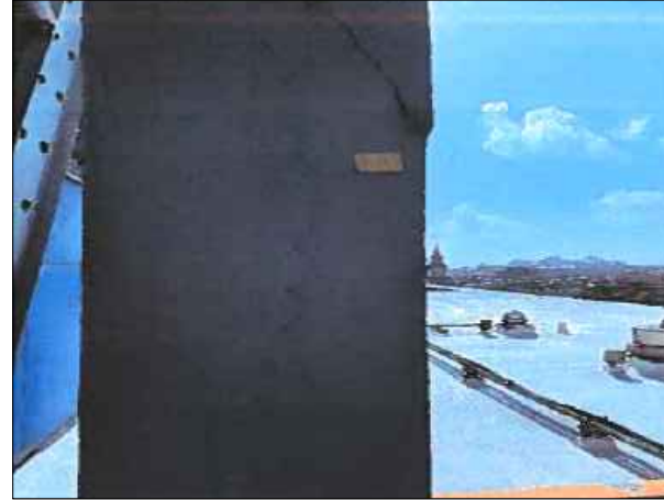
P5 ROOF COLUMN REPAIR
