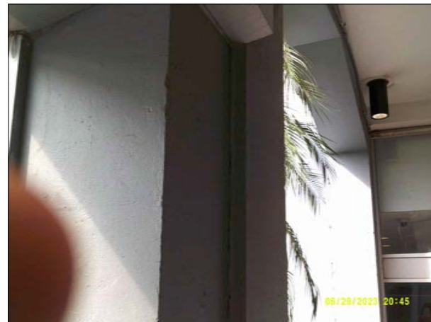
P7 GROUND LEVEL REPAIR
