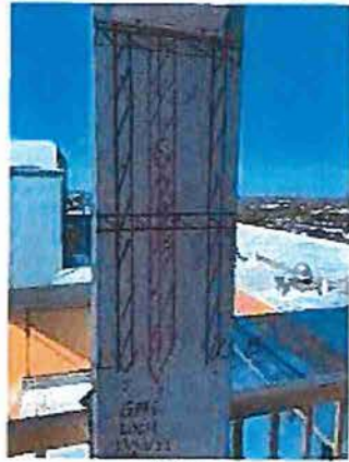
Loc. 4 Typical Rebar Pattern
