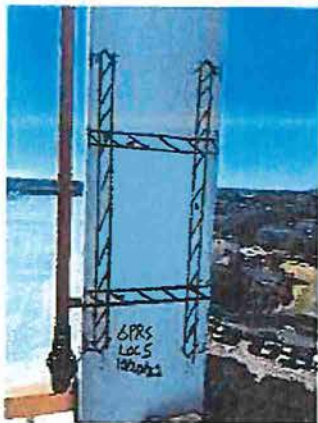
Loc. 5 Typical Rebar Pattern
