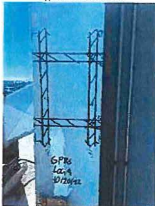
Loc. 9 Typical Rebar Pattern
