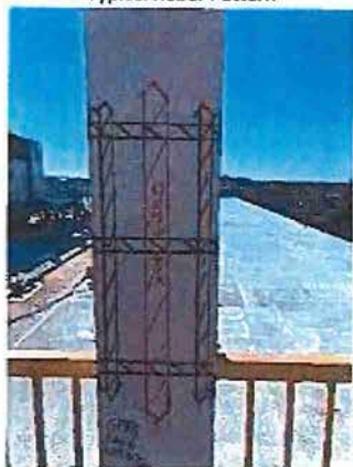
Loc. 6 Typical Rebar Pattern
