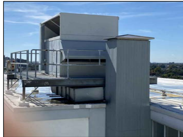
P14 VIEW OF STAINLESS STEEL CAP @ ANOTHER CHASE
