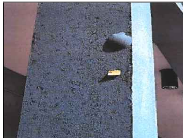
P8 GROUND LEVEL REPAIR
