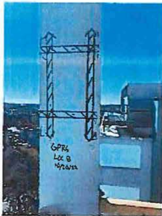
Loc. 8 Typical Rebar Pattern
